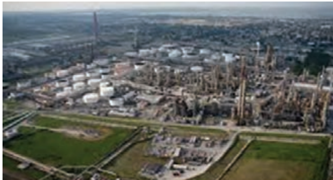
Fig.9: A chemical plant
